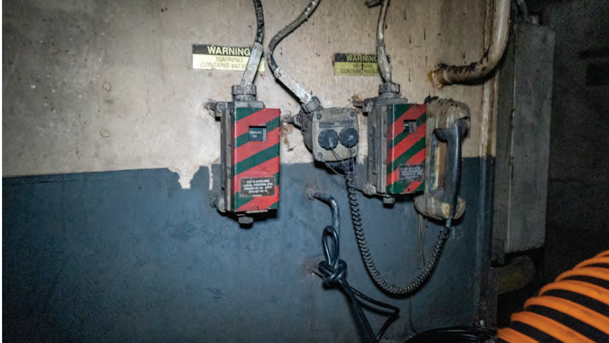
Figure 31, Still photo of AFFF push-buttons for sprinkler groups 15 and 16 serving Lower V with covers closed (16 on left; 15 on right). These push-buttons are in Upper V amidships.
