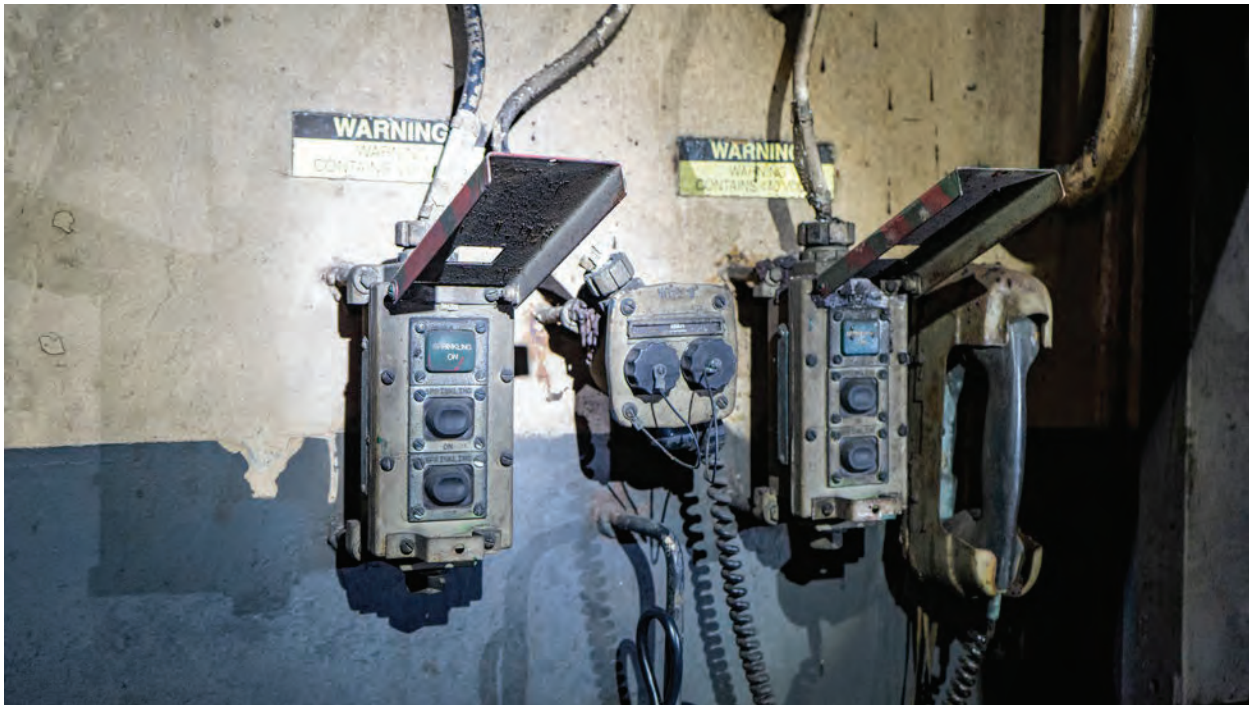
Figure 32, Still photo of AFFF push-buttons for sprinkler groups 15 and 16 serving Lower V with covers open (16 on left; 15 on right). These push-buttons are in Upper V amidships.
